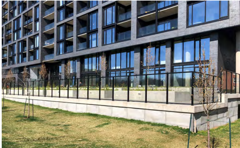
Grade-level separation between private outdoor space, and the public Gorsebrook Park are designed to capitalize on park views for residents.
