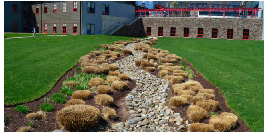
An example of an on-site swale and rain garden system (Source: Montgomery County Planning Commission, Flickr)
