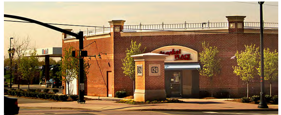
A gas station with a convenience store in front and pumps in the back creating a more amenable environment for pedestrians (Source: Brett VA, Flickr).
