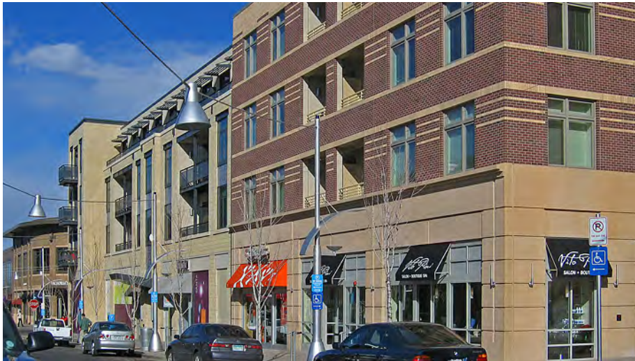
Consistent sign placement integrates into the overall facade composition. (Source: Brett VA, Flickr)
