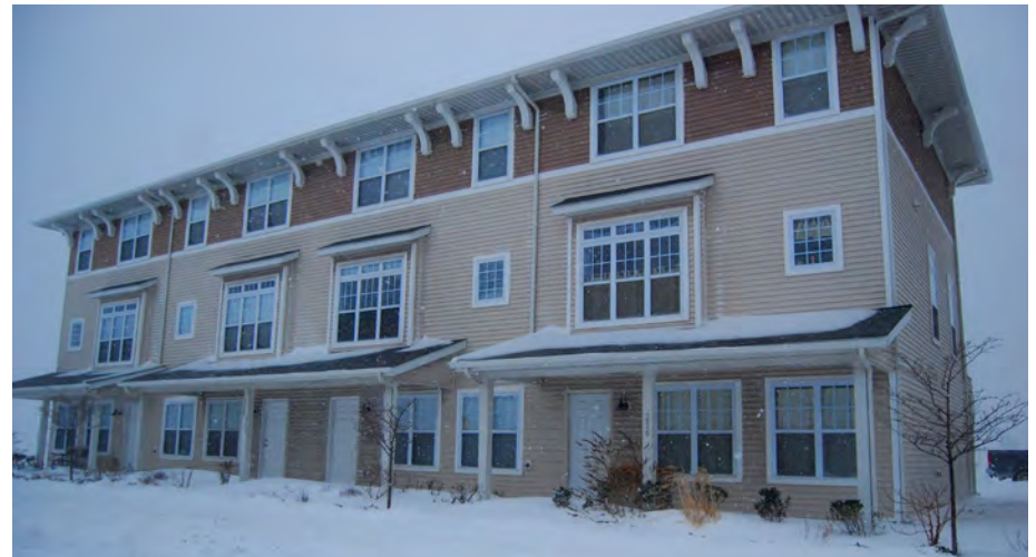
Townhouse Development with significant porch features and roof treatment. (Source: Rona Proudfoot)
