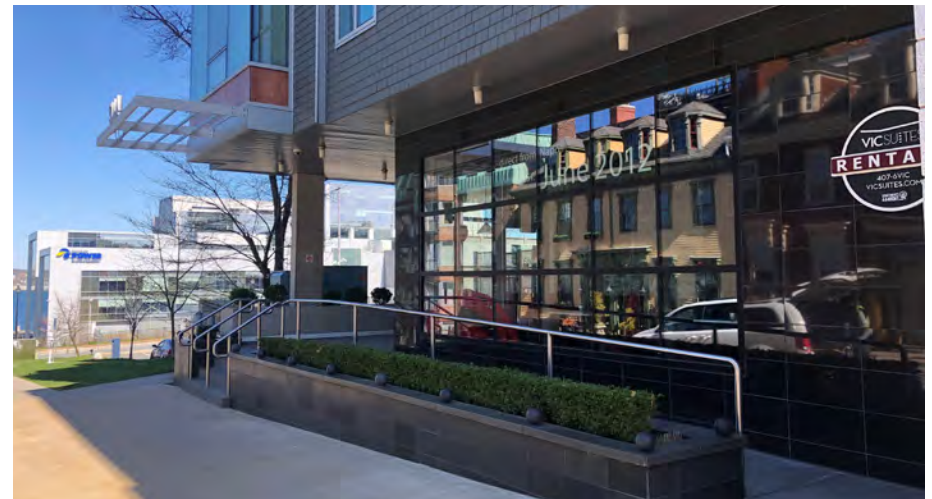
The VIC building (Halifax) combines articulation, landscaping, and transparency create an interesting building for pedestrians.
