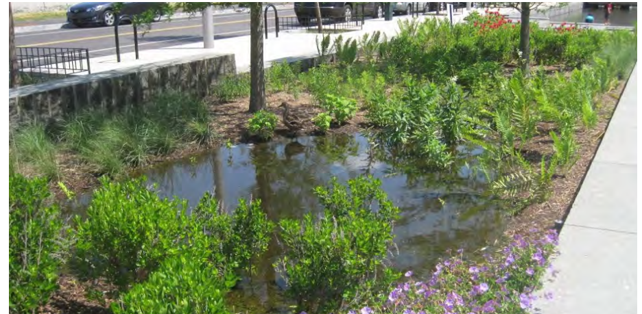
Rain Garden example located within the street right-of-way, acting as a green sponge for rainwater, and offering a reminder for pedestrians to natural systems.
