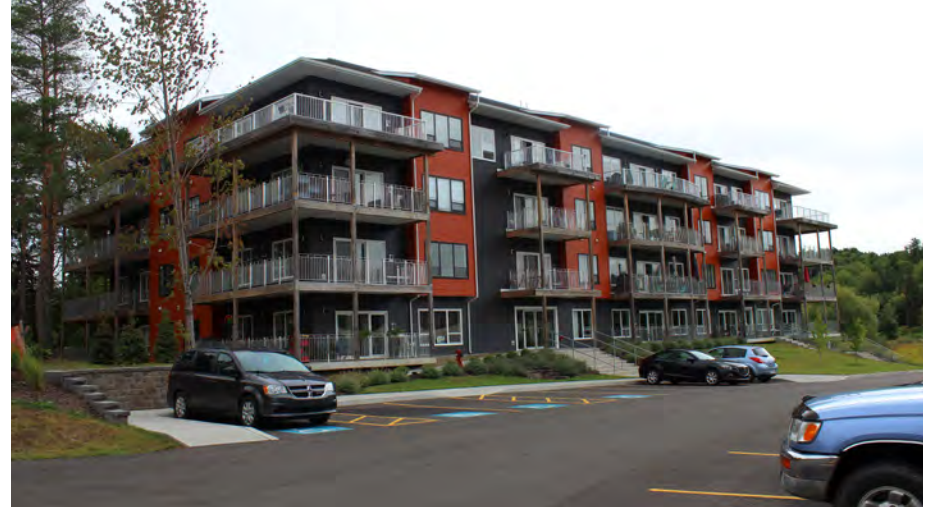
New multiple unit dwellings incorporate larger, more useable porch spaces, and are generally clad in vinyl or metal siding and under four storeys.
